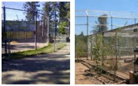
Compliant big cat fencing
